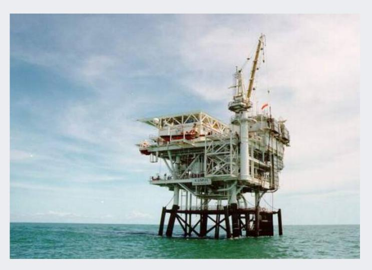
Fibre connection to a fixed offshore platform (Kumul Marine Terminal) through a J-tube. Provides communication from the platform and associated equipment to Port Moresby
